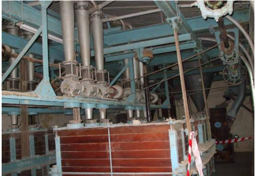
Underground emergency Flour Mill
